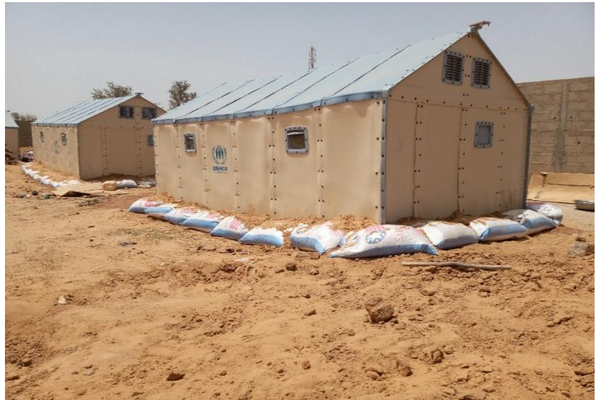
In Burkina Faso, RHUs were built to provide sturdier homes to IDP families affected by the heavy rainfalls and the floods in Wendou in the Sahel Region. ©UNHCR / S. Tchagbele
