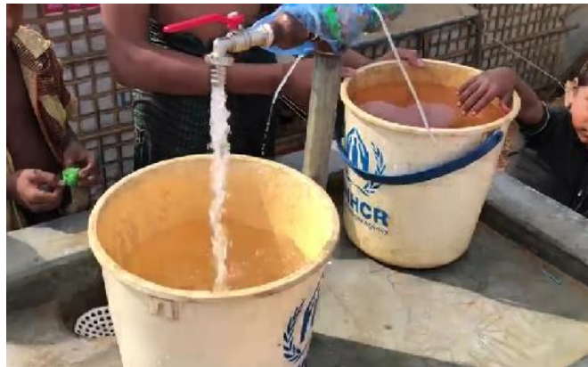
Chlorinated water tap that has started operating in Kutupalong with the support of UNHCR's water, sanitation and hygiene
