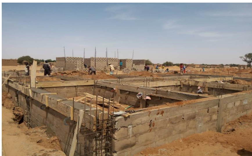
Construction site for the Integrated Health Centre Type II in Abala
