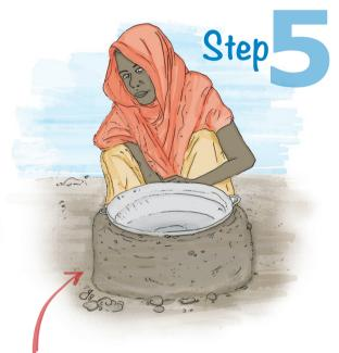
Build a 4 cm thick clay wall around the bricks until level with the top of bricks. The outer side of the bricks are to be slightly embedded into the wall.
