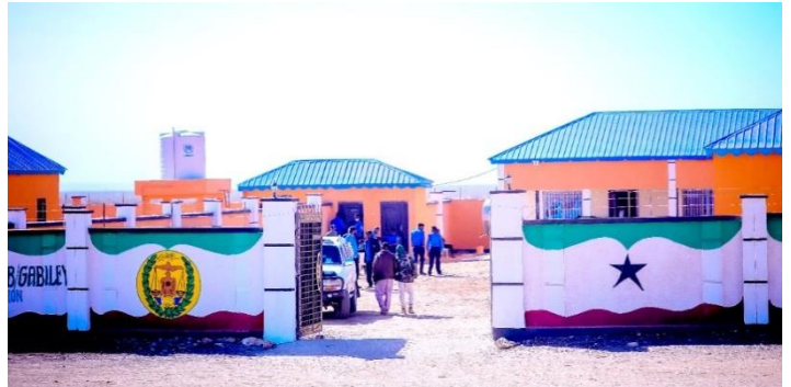
Newly constructed immigration center in Wajaale. © UNHCR
