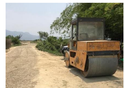
Road project, before and after compaction, Maungdaw. Photo:
