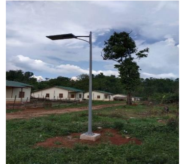
Installation of solar streetlights, Kayah State. Photo: UNHCR
