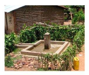
Figure 8. 1: A Well constructed and maintained tap stand in Kabarole
