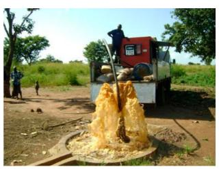
Picture 5. 6: Borehole blowing/cleaning in Pader
