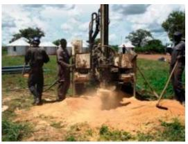
Picture 6. 7: Air percussion drilling with a light PAT 401 rig in Nwoya district
