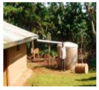
Picture 6. 12: Ferrocement Tank (4m³) in Kapchorwa
