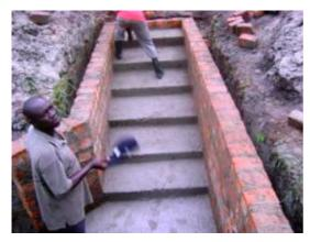
Picture 6. 3:Spring construction in Oyam
