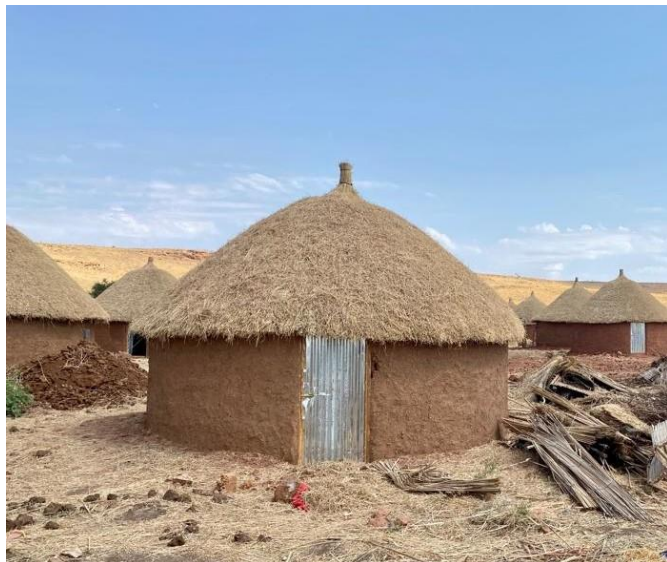
To date, 175 tukuls (durable shelters) have been completed in Um Rakuba © UNHCR
