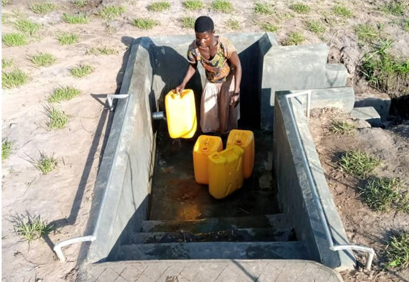
Completed spring in Pajulu sub county – Arua district
