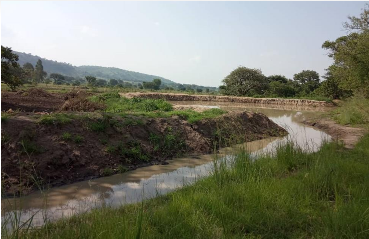
Water pond constructed during resilience design in Nebbi district
