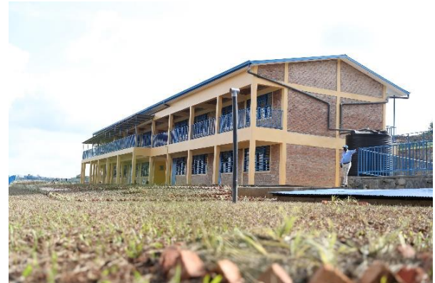
Newly constructed 16 classrooms in Kigeme, Nyamagabe District @UNHCR/Eugene Sibomana
