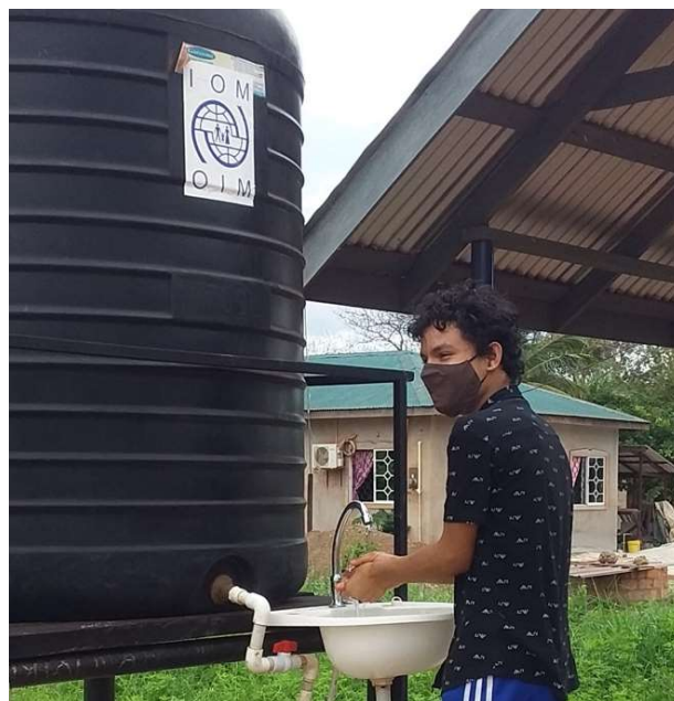
June 2020 Set Up of Hand Wash Stations
