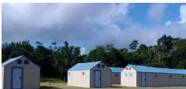
Refugee Housing Units transformed into medical and quarantine facilities in Moruca
