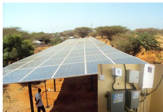
Photovoltaic modules and solar power inverter at borehole in Hagadera
