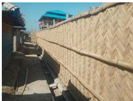
Fencing constructed around a quarantine centre in Camp 4 Extension in the large Kutupalong settlement. ©UNHCR/Ciobanu, I
