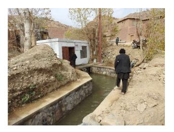
The project involves the construction of a Micro Hydro Power (MHP) plant with an intake, 300 metre feeding canal, forebay, penstock, power house with turbines and gridlines to individual households.
