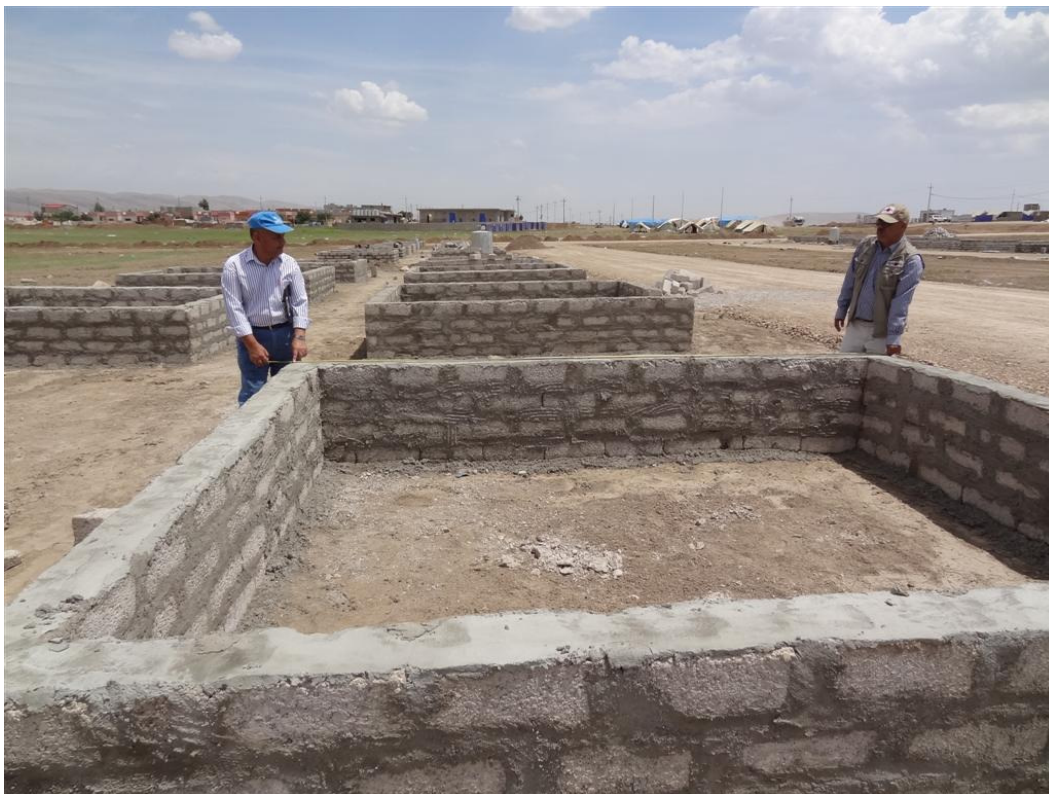
Construction of walls and casting foundations of tents
