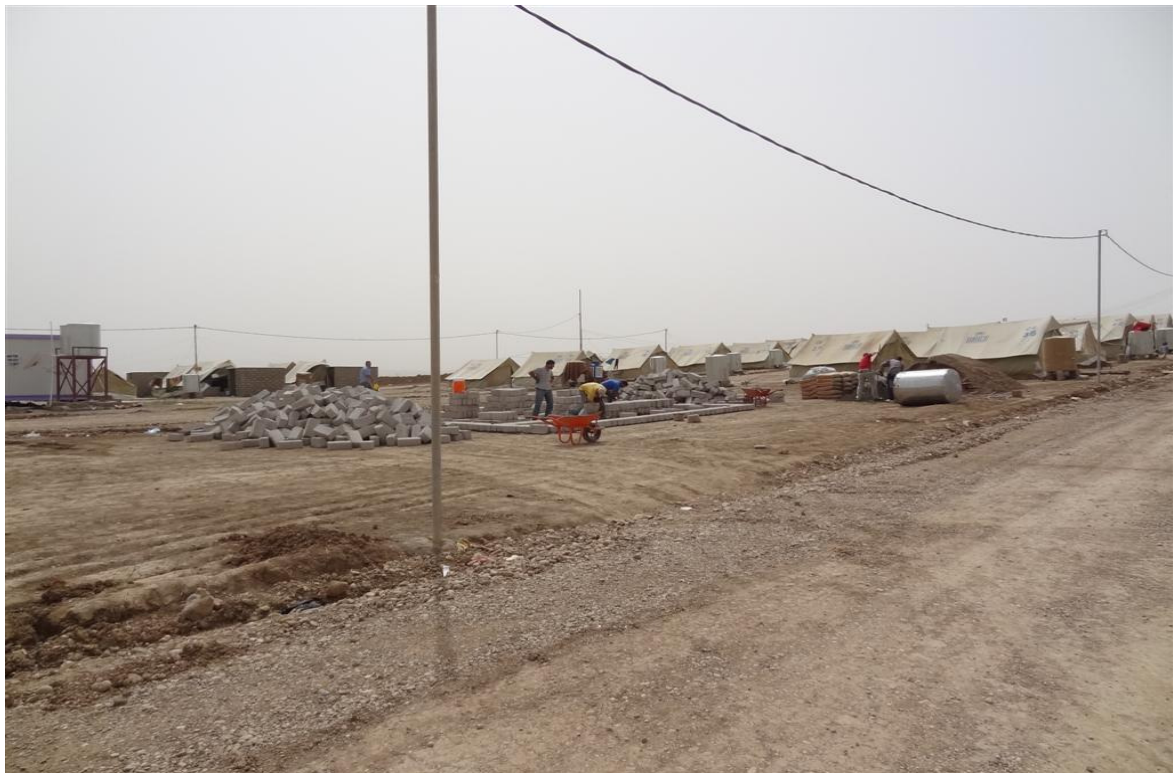
On going procedures of construction in Domiz Camp
